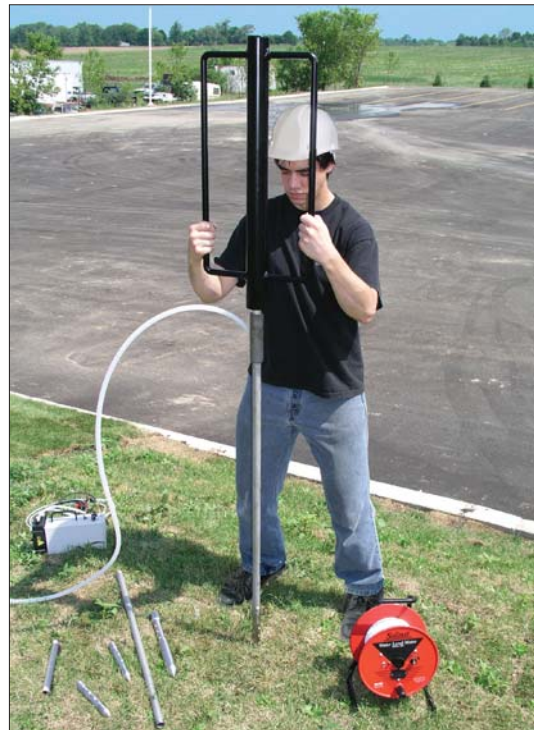
Installing Piezometers with a Manual Slide Hammer
